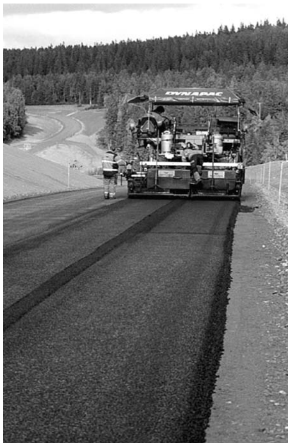
FIGURE 11.12 Paving of semi-dense cold mix asphalt.
